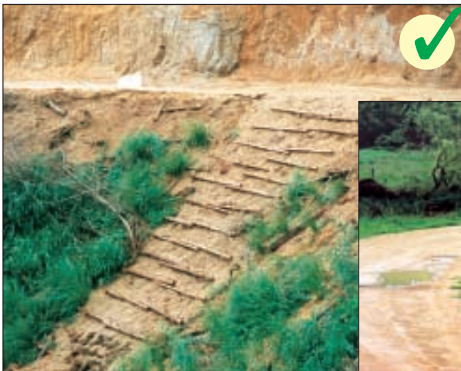
Effective embankment protection reduces road maintenance costs
