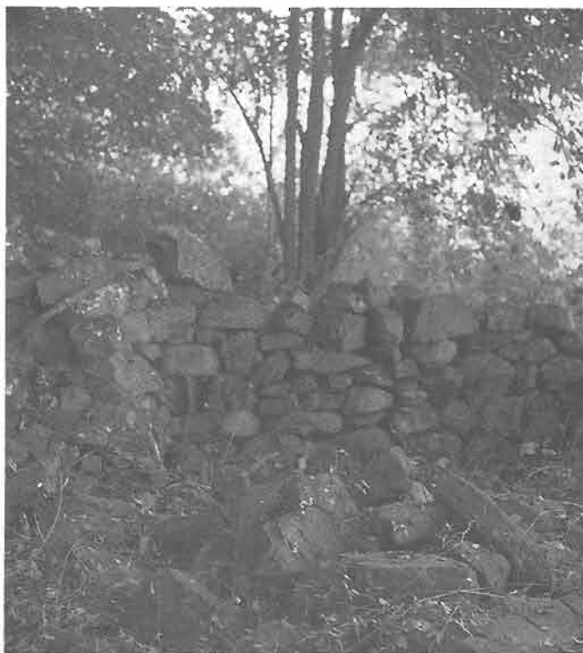
Above, below and right: Ruins of zebra stables constructed of massive stone walls, at Beestekraal
