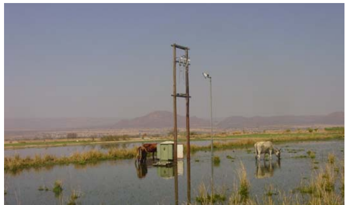
Figure 17: Waste water evaporation ponds in Sekhukhune District, Limpopo
