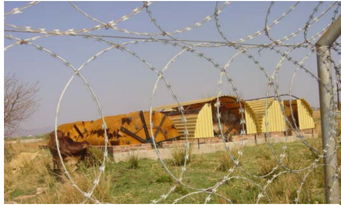
Figure 16: Sewer treatment plant in Sekhukhune District, Limpopo
