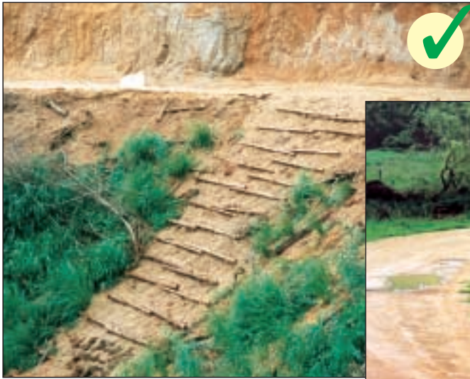
Effective embankment protection reduces road maintenance costs
